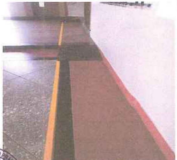
Ramp – Near Administrative Office
